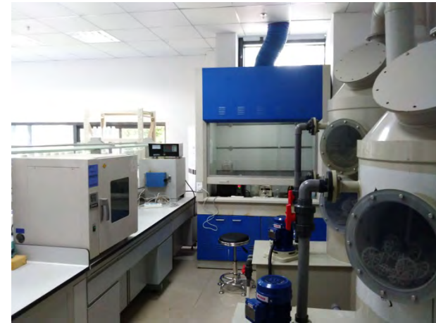
Air cleaning unit
